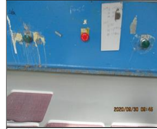
Photo of the inside of the main production hall Two hands operate devices.JPG
