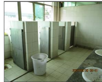
Photo of the sanitary facilities Toilets.JPG
